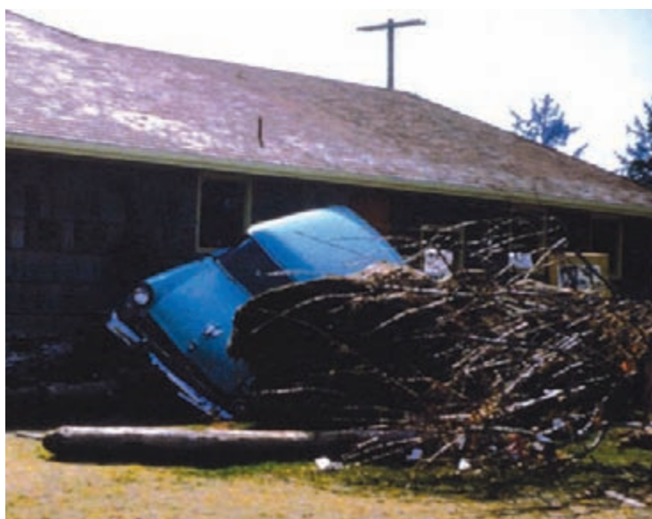
Destruction at Seaside, Oregon, due to the March 28, 1964, Alaska tsunami. Water lifted the car against the house, uprooted the tree, and washed in driftwood logs. Beach grass hanging in the tree branches indicates the maximum water depth at this location was 3.5 m (12 ft). This house was 1200 m (4000 ft) from the shore. (Photo source: Herb Schlappi)
